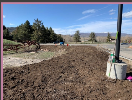
Day of restoration 2020
